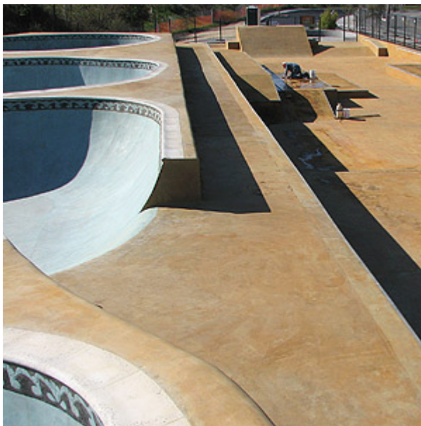
The skate park is the first to have every concrete surface colored with acid stain.
